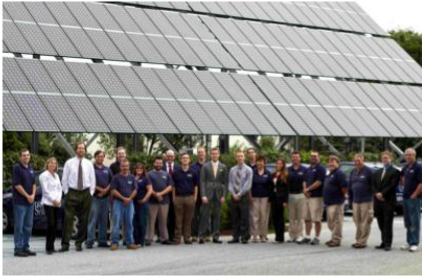
Haverford Systems is 100% Solar Powered.
